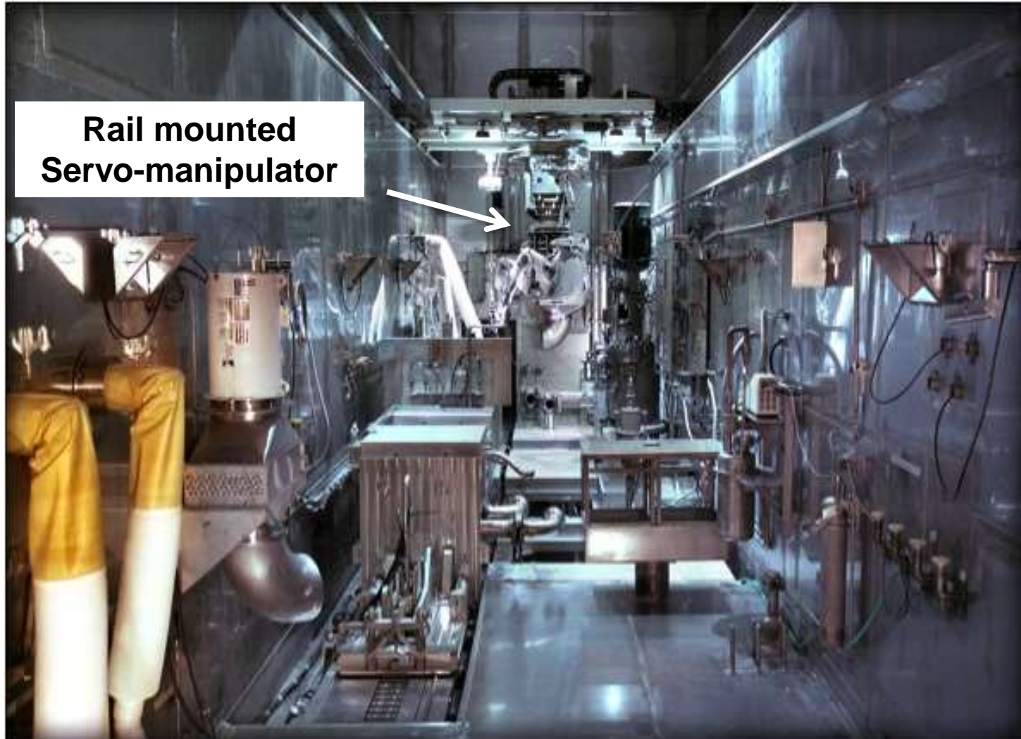
View of the Service Bay Looking West
