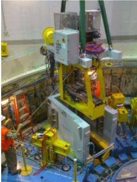
Installation of CVI Robot
