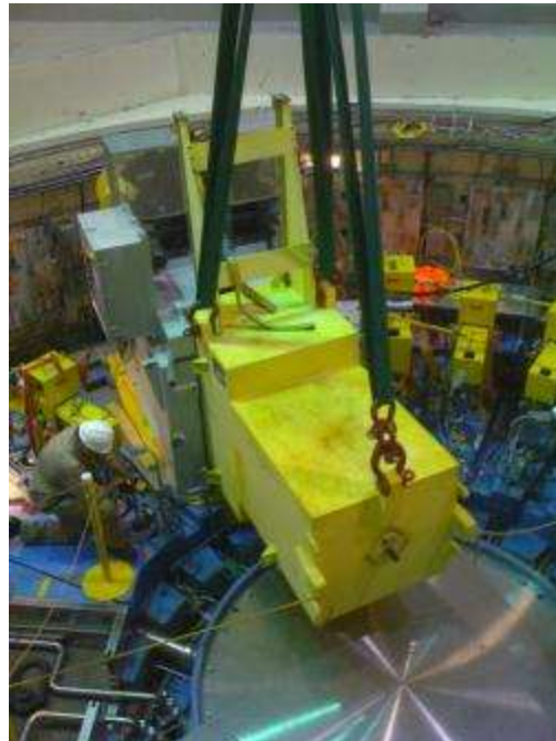
Installation of CVI Plug Cask
