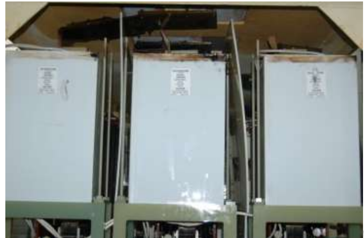
New capacitors failure (brackets removed)
