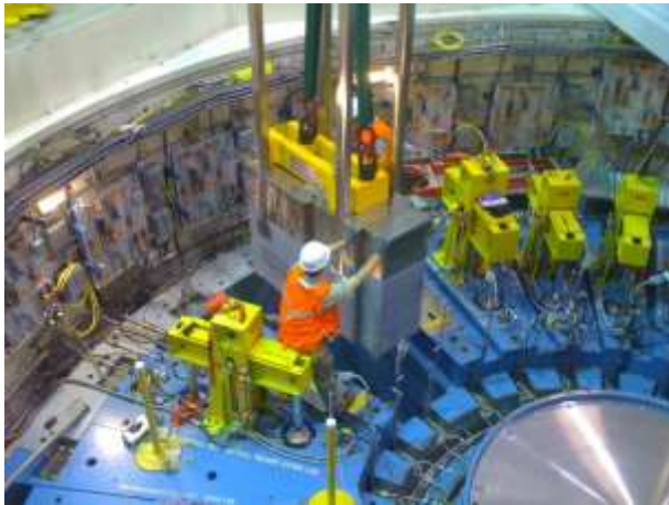
Lower Segment Installation (31,000 lbs/14,000kg)
