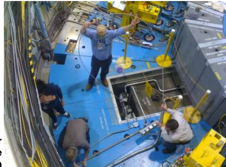
TIS Fiber Optic Cable Installation
