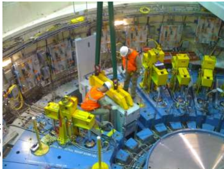
Middle Segment Installation (20,000 lbs/9100kg)
