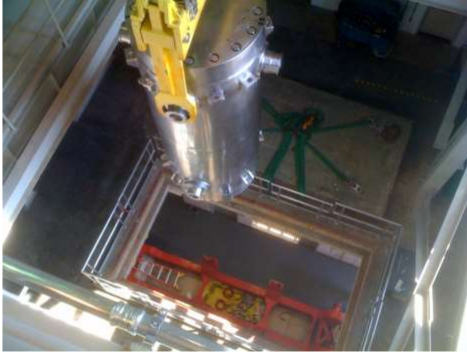
Cask Lifting from Truck
