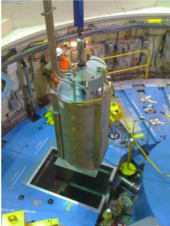
New PBW Installation
