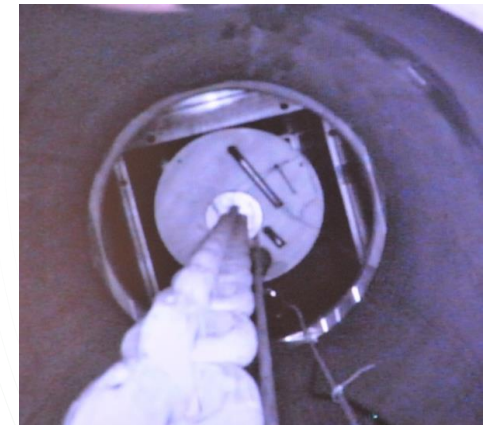
PBW Being Pulled into Cask
