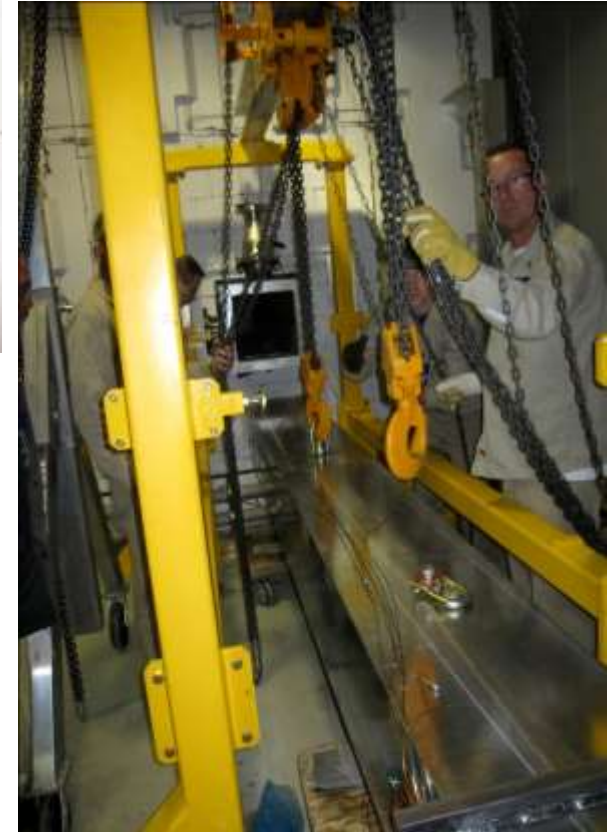
Beam Stop Vessel Installation
