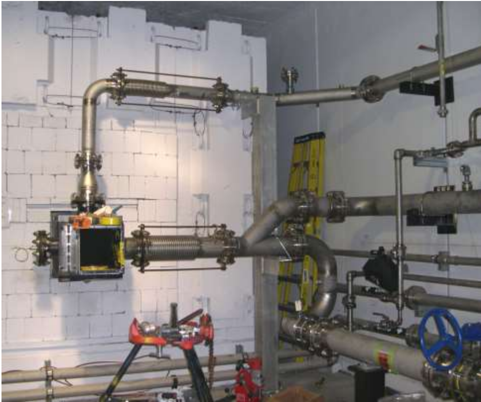
Cooling Loop Installation looking at Dump
