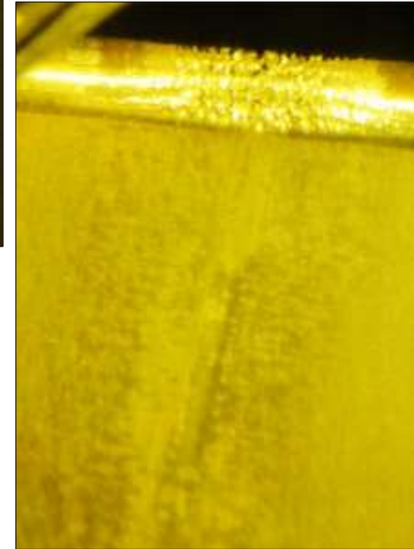
Center Baffle (after cleaning)
