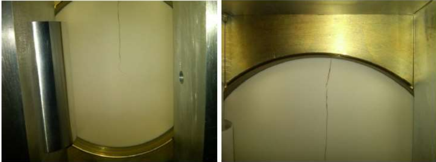
Figure 3 - CCL Window with fracture of ceramic window.
