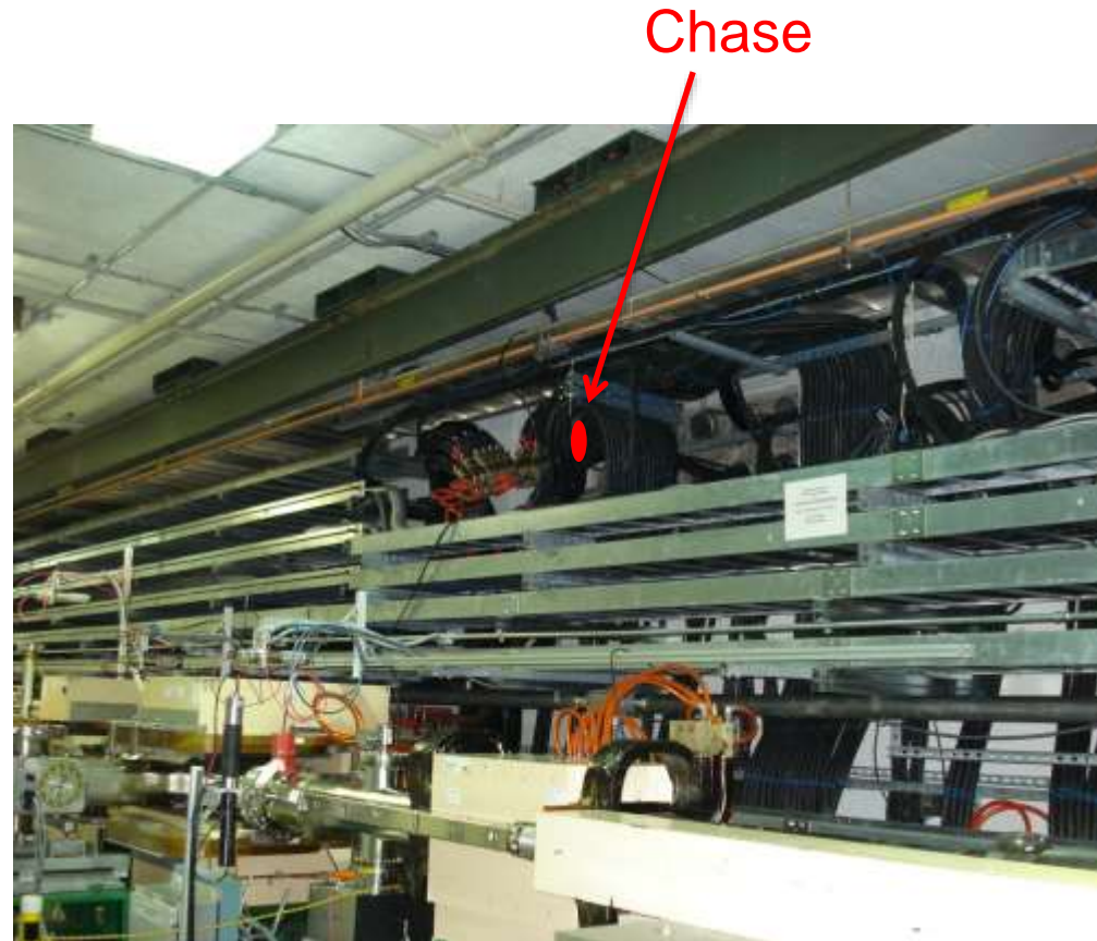
Photo of ring injection area
