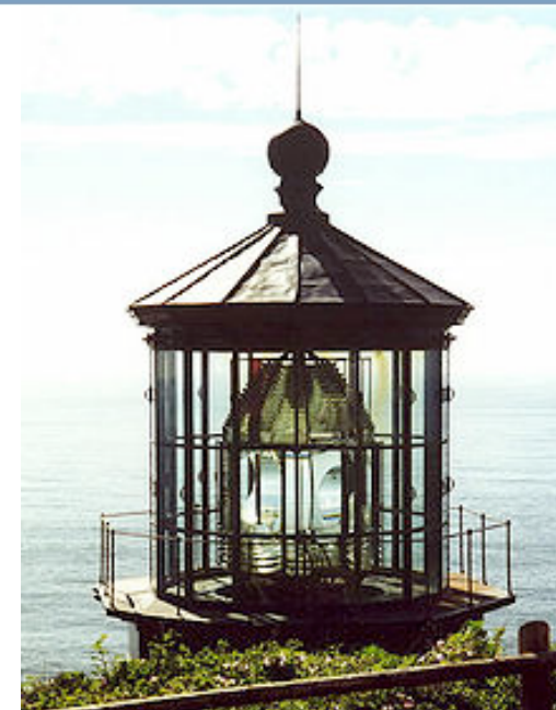
Cape Meares Lighthouse (Oregon); first-order Fresnel lens
