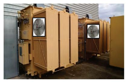
Figure 5.12. Photo of the main ring dipole power supply substation transformers with cooling fan images superimposed.
