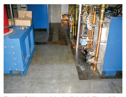
Figure 4.41. Existing ground-plane installation in the Klystron Gallery.
