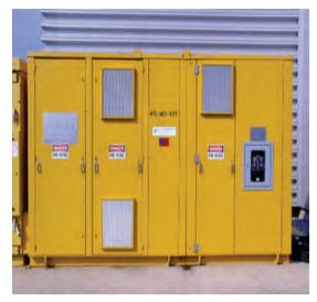
Outside 13.8 kV:2100 V 1.5 MVA transformer
