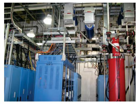
Figure 4.40. Existing cable tray in the Klystron Gallery.
