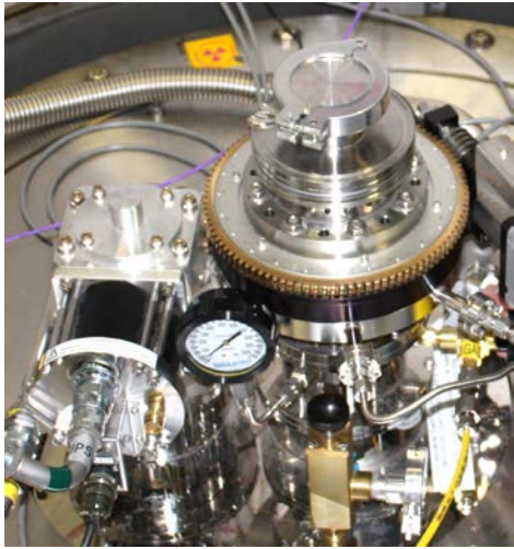
Figure 5. Flange blank in place on the cryofurnace
