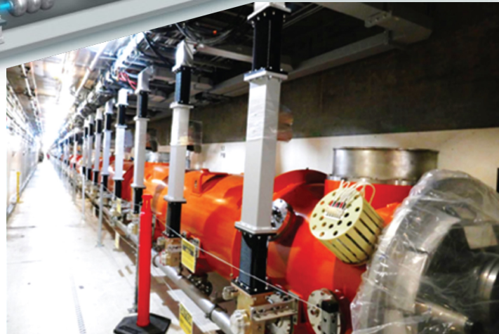
All cryomodules installed and welded
