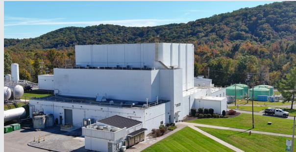
**HFIR uses uranium-235 as the fuel to generate the highest rate of flowing neutrons, or neutron “flux,” available for research in the United States.**
