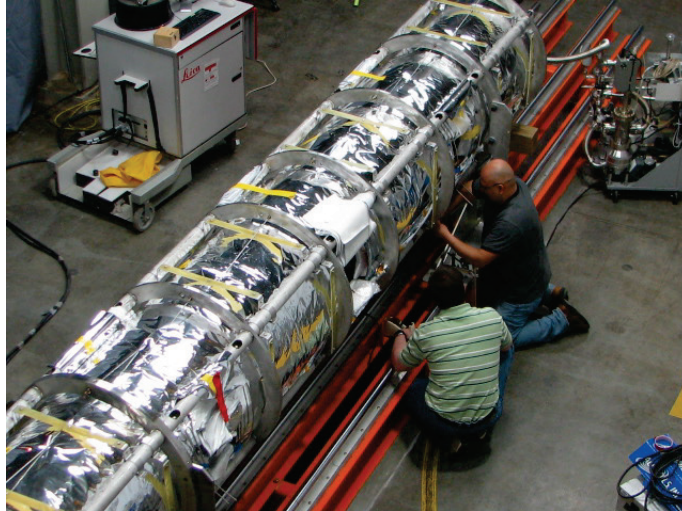
Figure 3.13. Cryomodule cold mass assembly.
